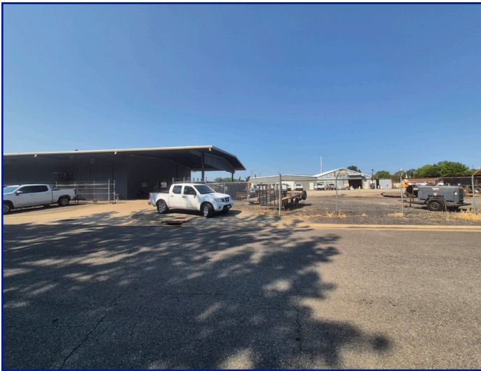
View of existing curb cut at southern property line
