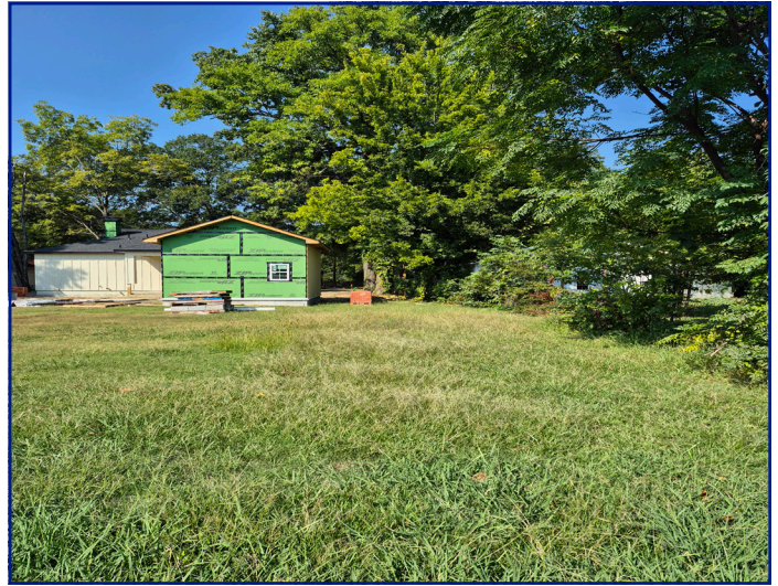
Rear side of outbuilding
