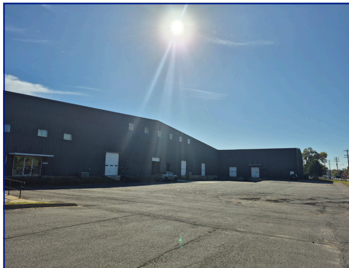
View of subject property facing SE
