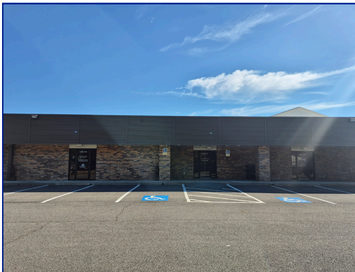
View of subject property facing E
