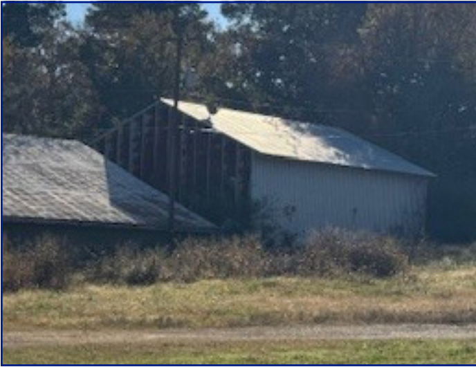
Building in setback
