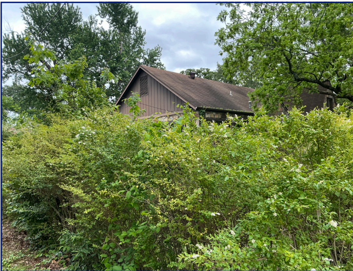
View of rear vent and aluminum siding
