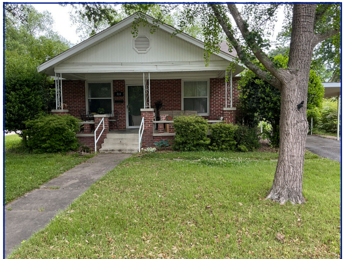
Property adjacent to the N
