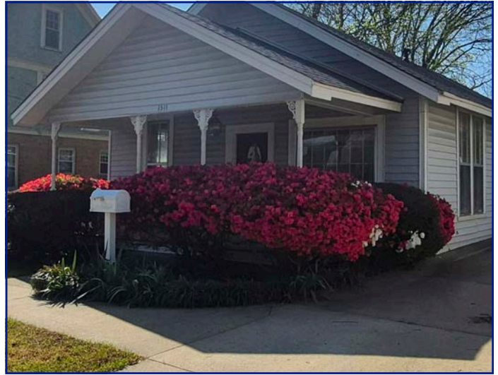
View of subject property facing SE
