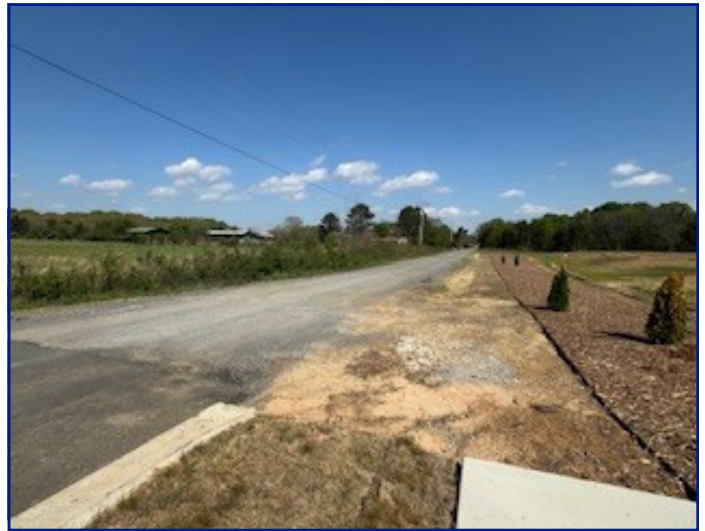
Current road improvement termination point
