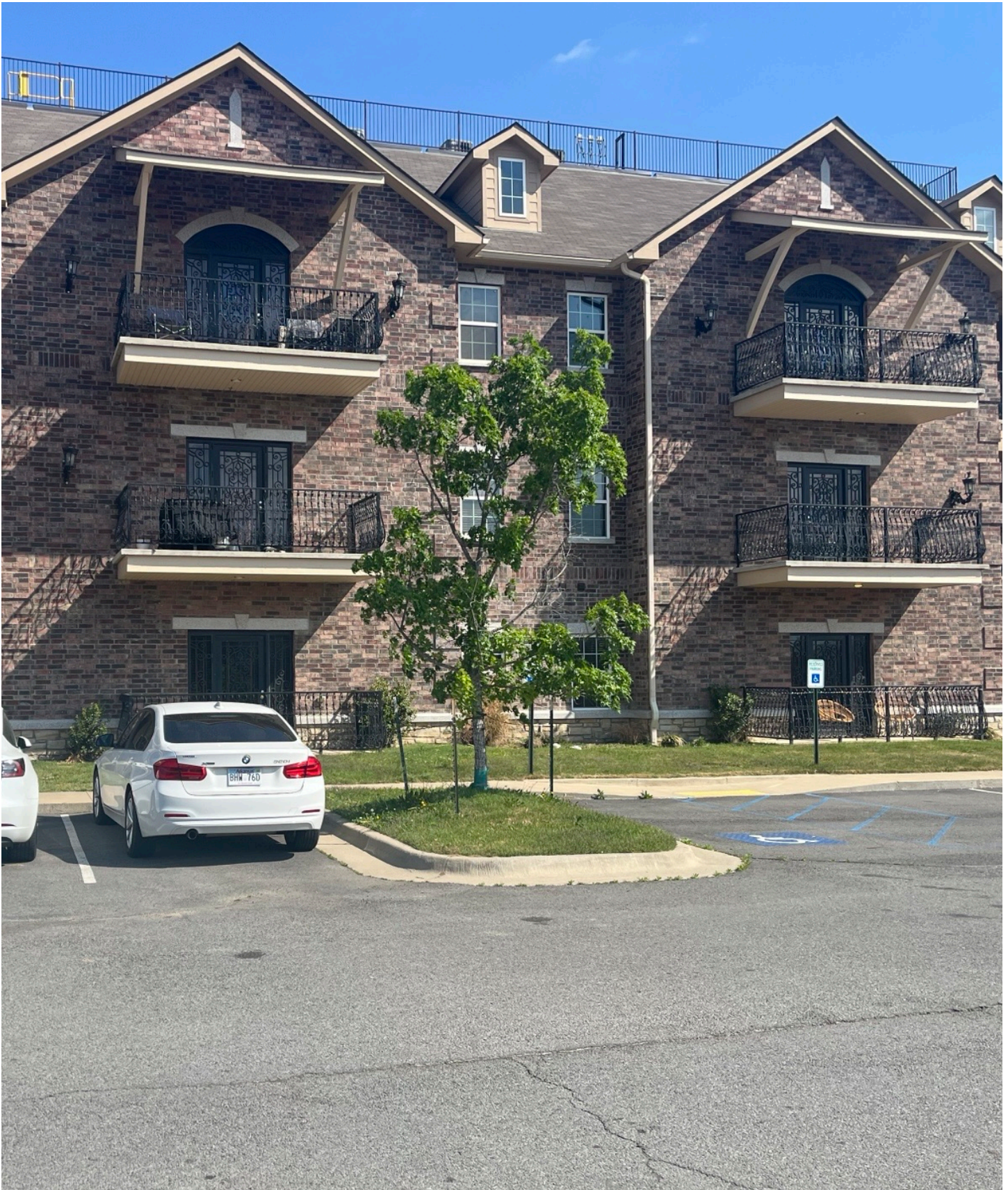
EXHIBIT G: As built Phase I
