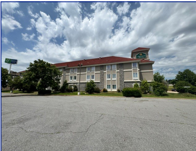
Property adjacent to the N
