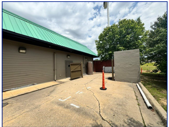
View of project location
