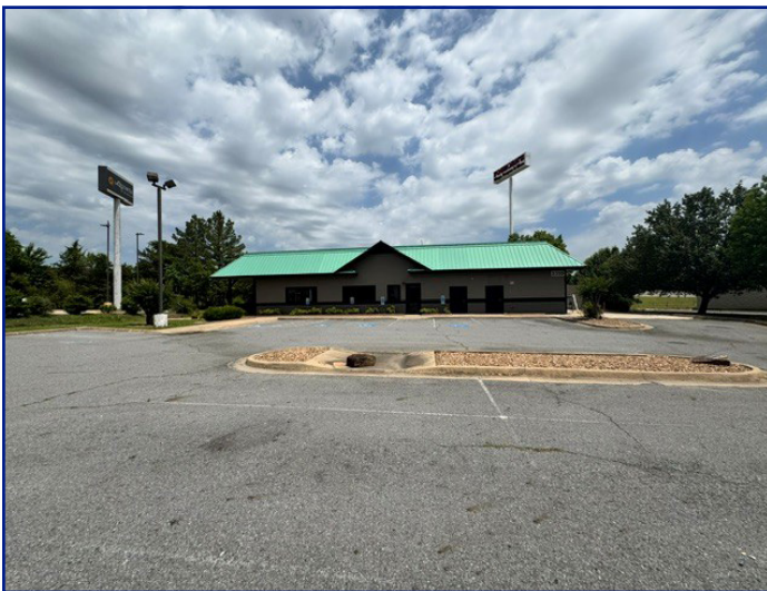
View of subject property facing E
